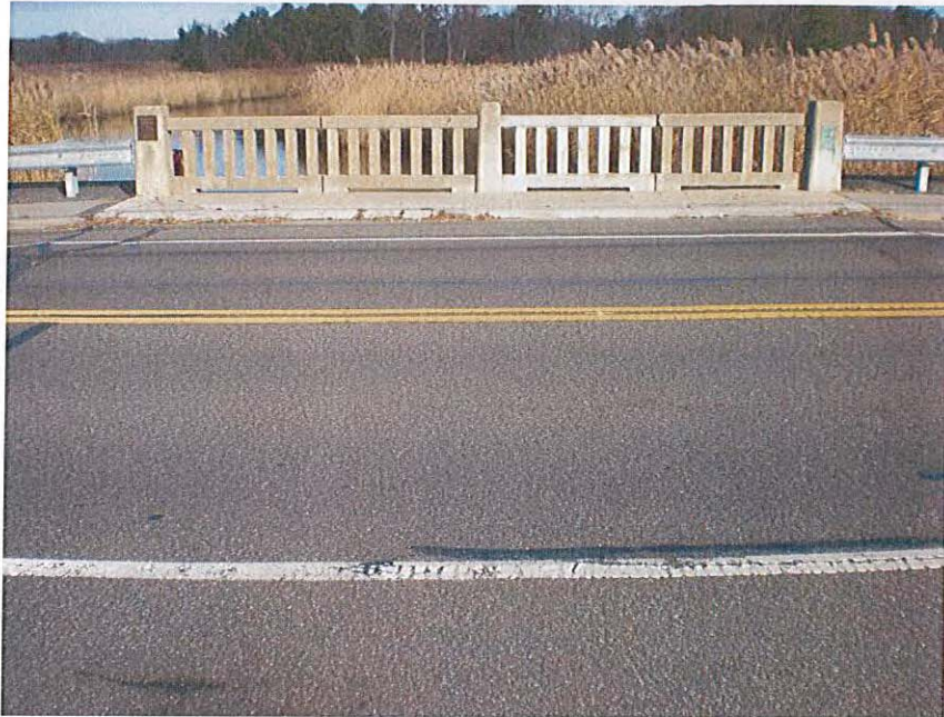
General view of bridge – looking north
