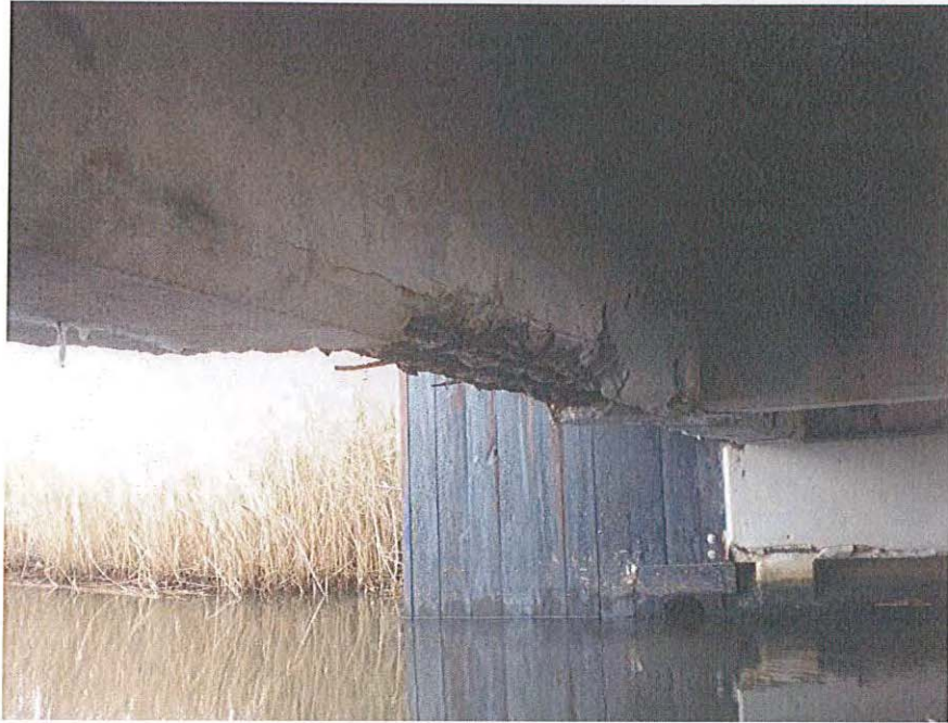
Fascia Beam A – Looking Northeast
