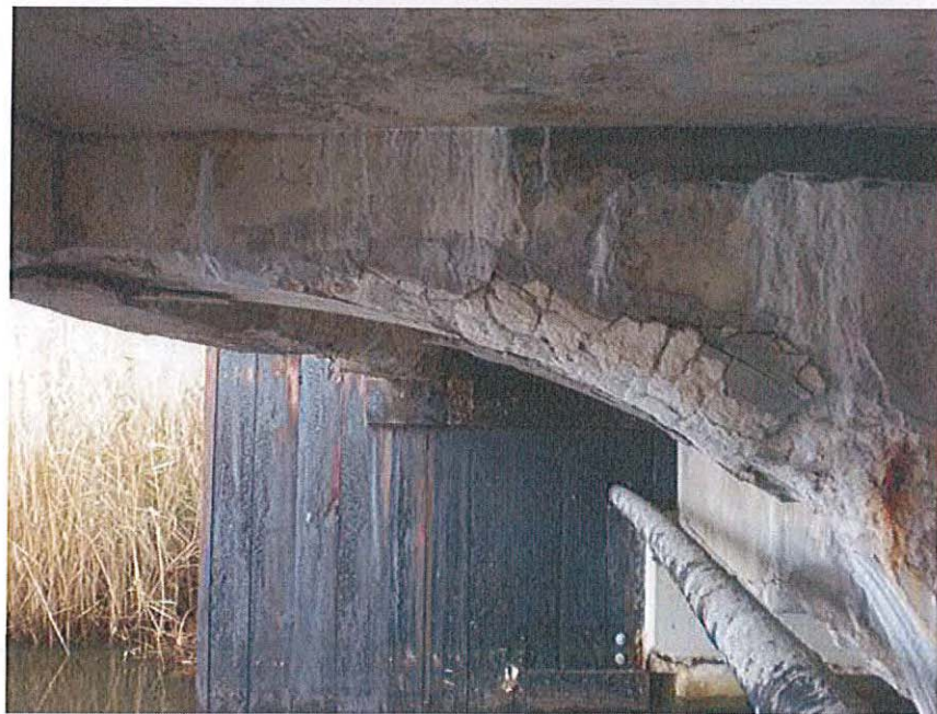
Sidewalk support beam – looking east – north side of bridge
