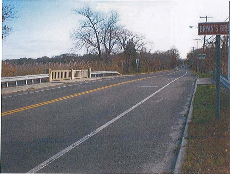
General View of Bridge – Looking East
