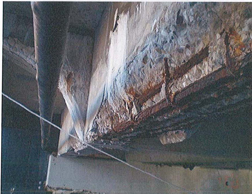
North fascia – Looking East
