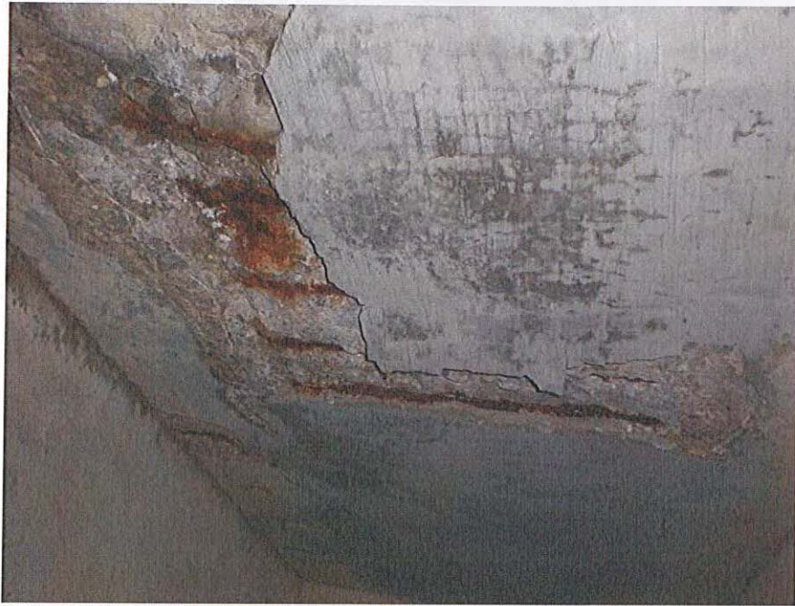
Between beams F and E - Looking East
