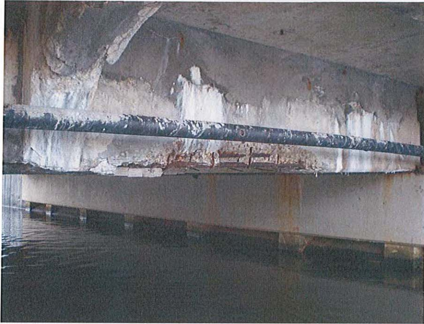
Fascia beam – Looking Southwest
