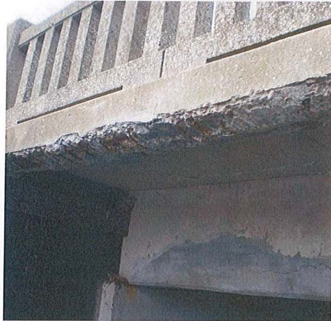
Parapet beam - South Side - Looking North
