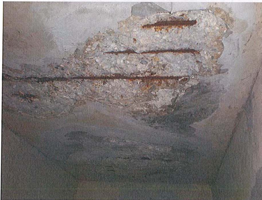
Bottom of Deck between D and E
