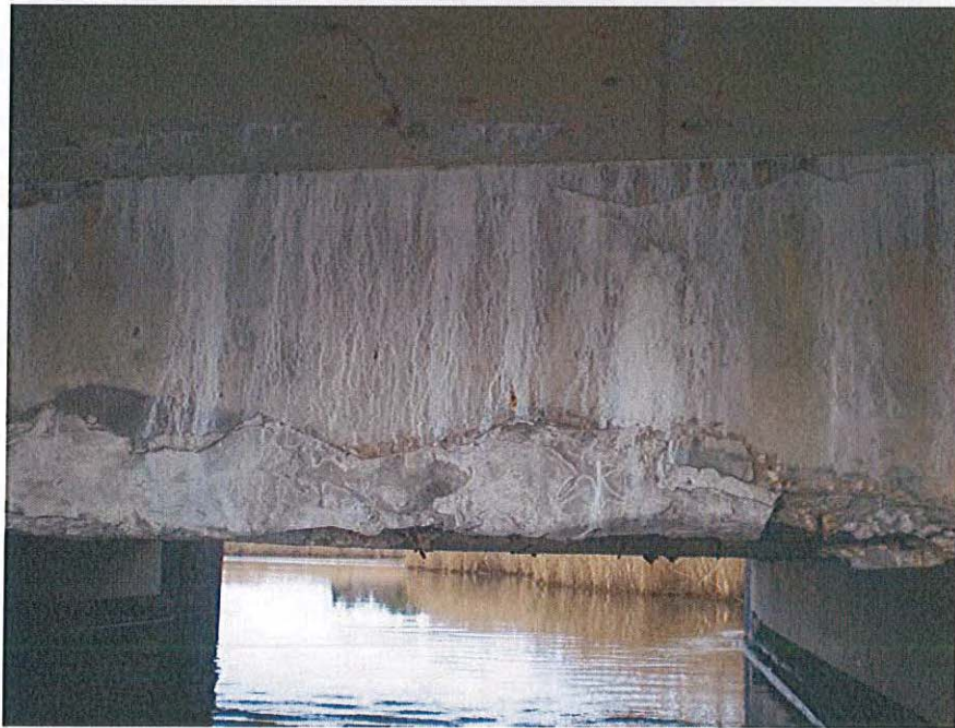
Fascia beam H – Looking North
