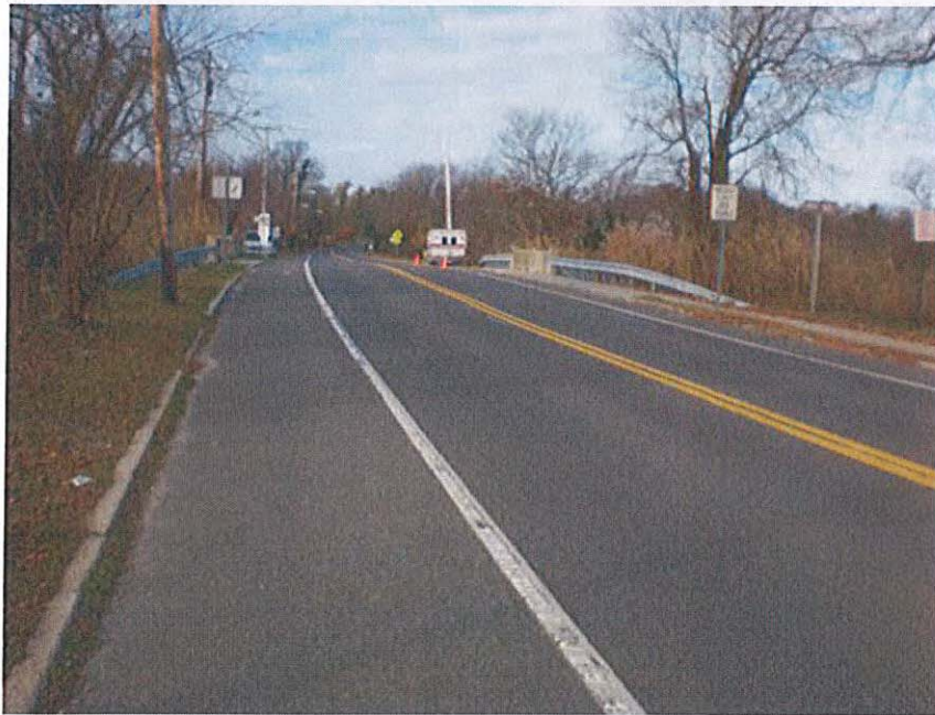
General View of Bridge – Looking West
