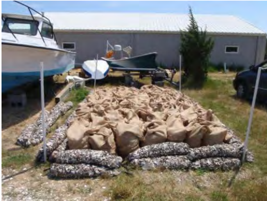
Mock-up of a 3 by 5 meter reef with perimeter bags (G. Rivara photo).
