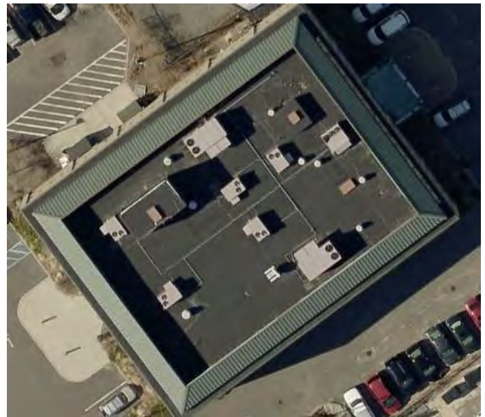
Figure 37: Roof of Cornell Coop. Ext.
