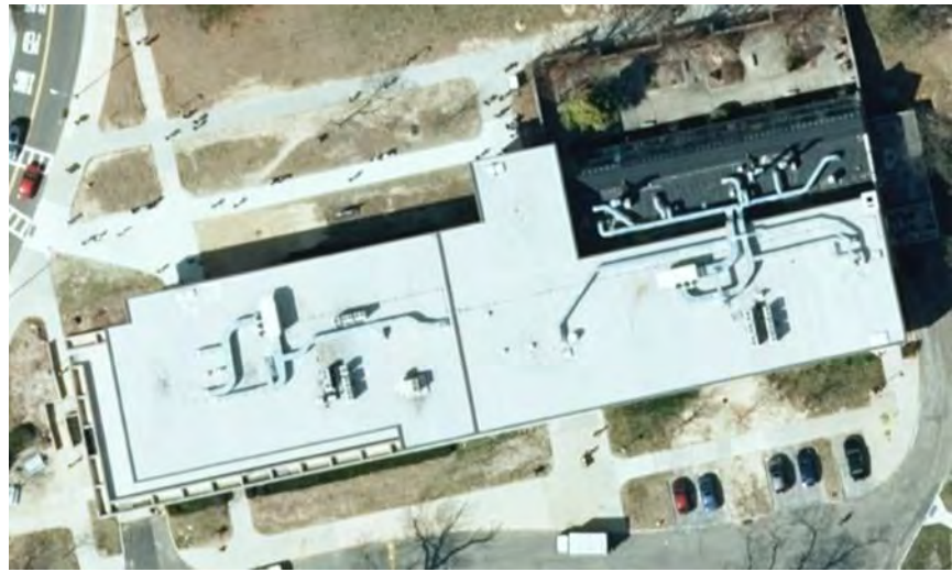
Figure 16: Roof of Southampton Building.
