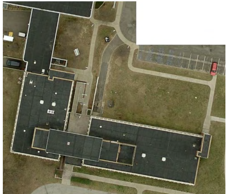
Figure 23: Roof of District Attorney Roof.
