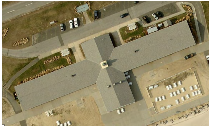
Figure 38: Roof of Pavillion.
