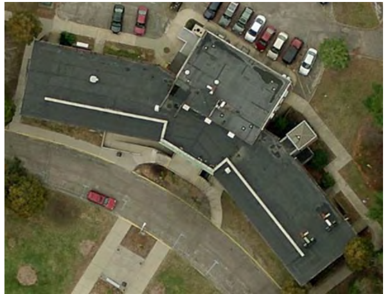
Figure 10: Roof of Kreiling Hall.
