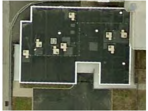
Figure 3: Roof of Day Care Center
