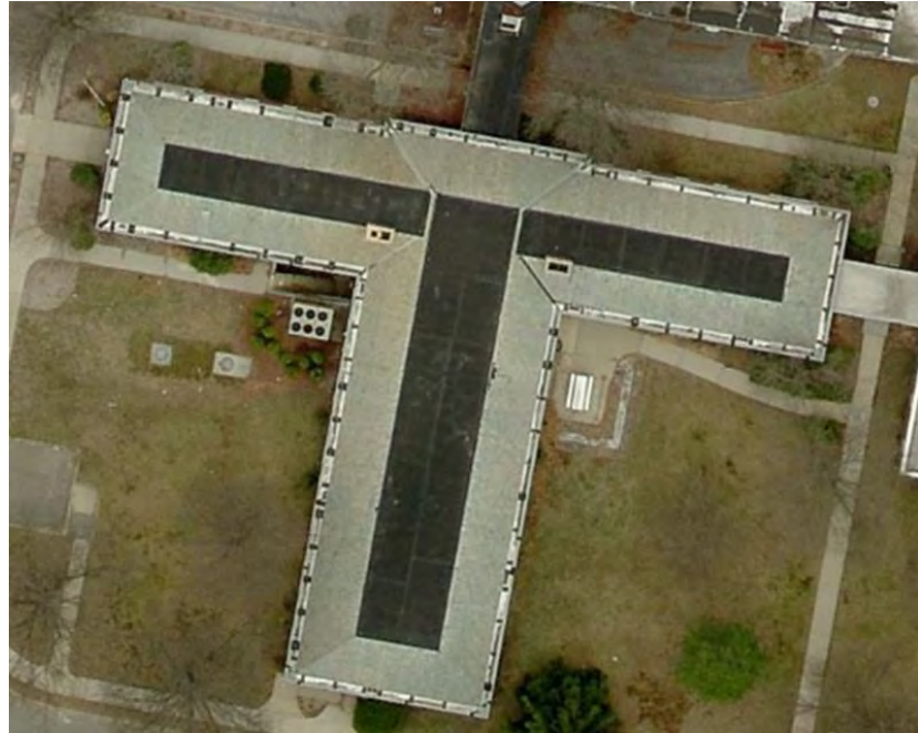
Figure 25: Roof of Labor Department.
