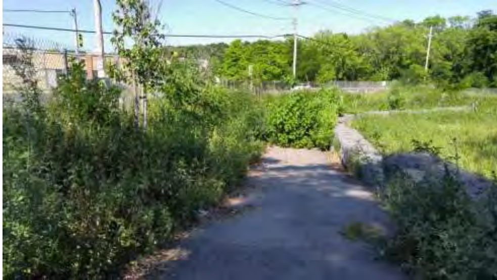
Photo 6: Recharge Basin Asphalt Driveway and Gabion Block Wall
