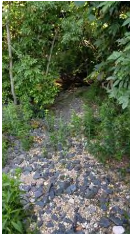
Photo 9: Riprap Leading to Swampawams Creek from Recharge Basin Property
