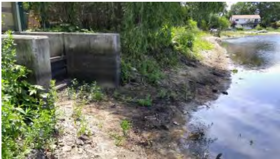
Photo 2: Concrete Weir Structure at South Bank of Deer Lake
