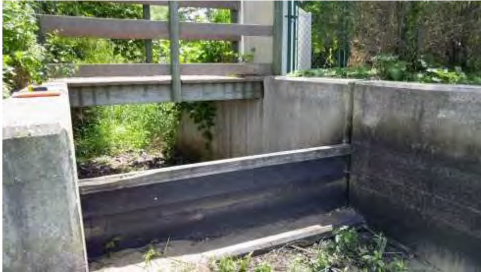
Photo 3: Concrete Weir Structure and Wooden Flashboard
