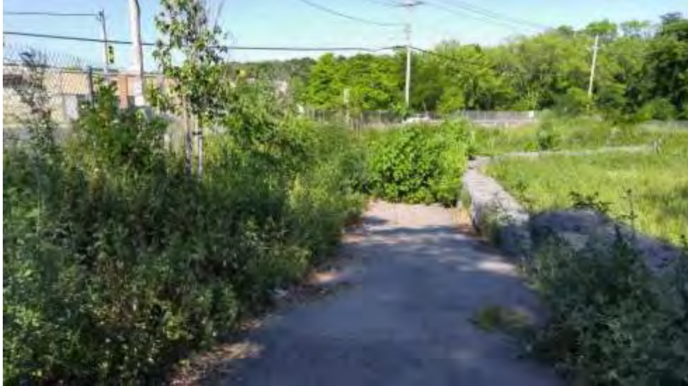
Photo 6: Recharge Basin Asphalt Driveway and Gabion Block Wall
