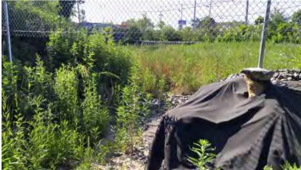
Photo 8: Recharge Basin Berm Opening, Partially Damaged from Storm Runoff
