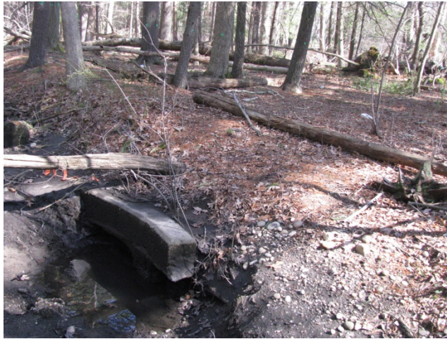
LOOKING NORTHEAST AT EXISTING HEADWALL SHOWING EASEMENT & ADJACENT AREA
