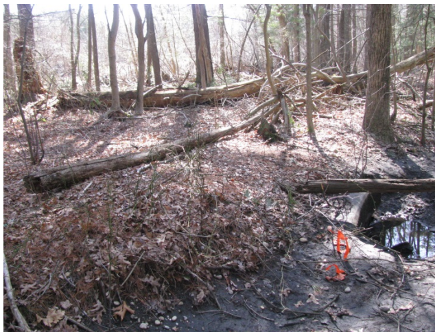
LOOKING SOUTHEAST AT EXISTING HEADWALL SHOWING EASEMENT & ADJACENT AREA
