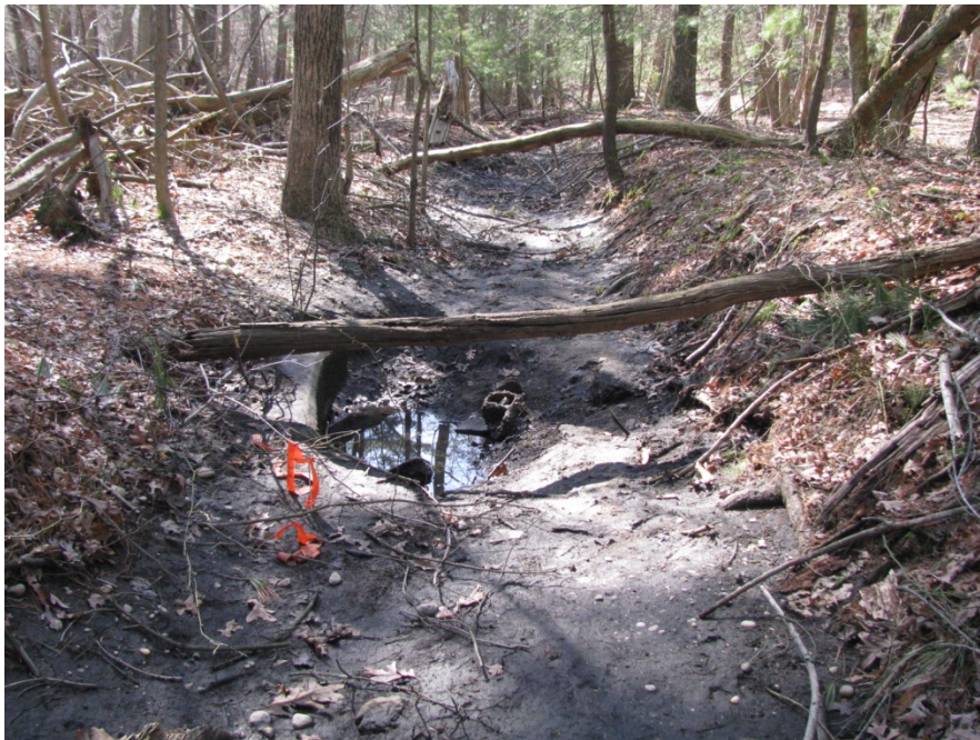
LOOKING SOUTH (DOWNSTREAM) AT EXISTING HEADWALL SHOWING CARMANS RIVER STREAMBED
